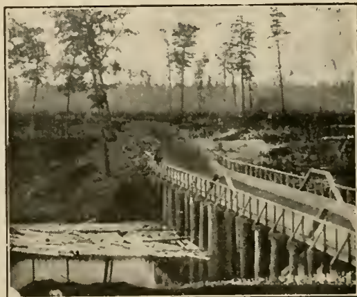
FIRST UNION STREET BRIDGE
